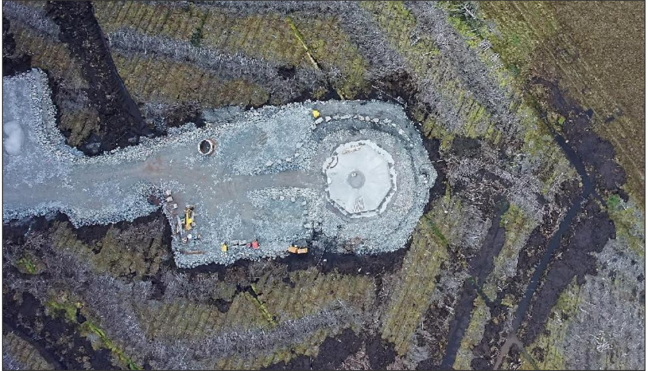
Figure 5.6: Minimising peat excavation through displacement construction methods.
