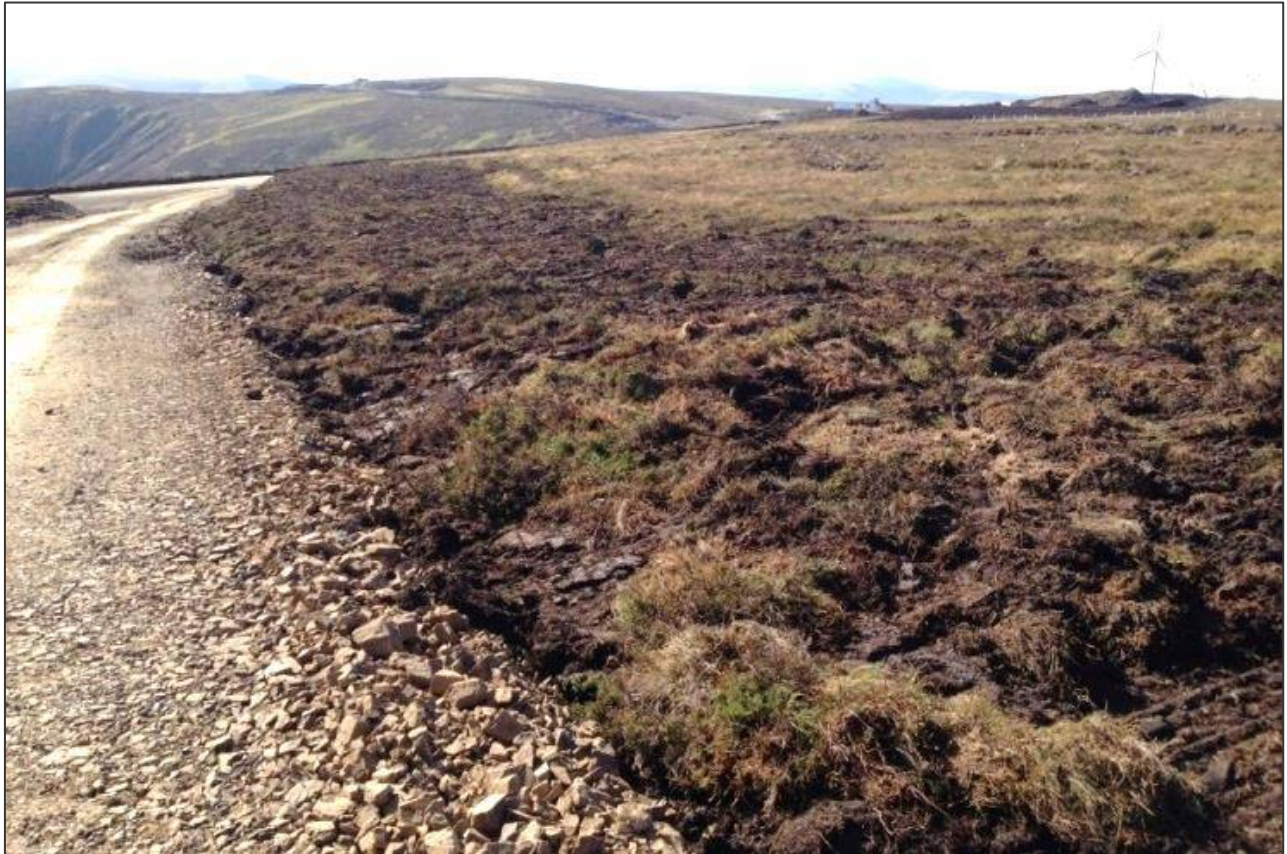
Figure 5.3: Example of access track verge reinstatement
