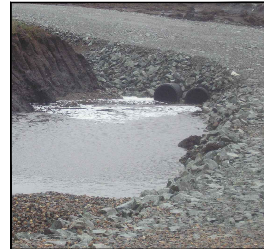
TYPICAL UNDER TRACK DRAINAGE
